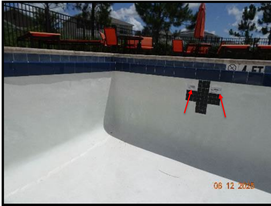
Photo 9 Additional view of past repairs to pool wall finish.
