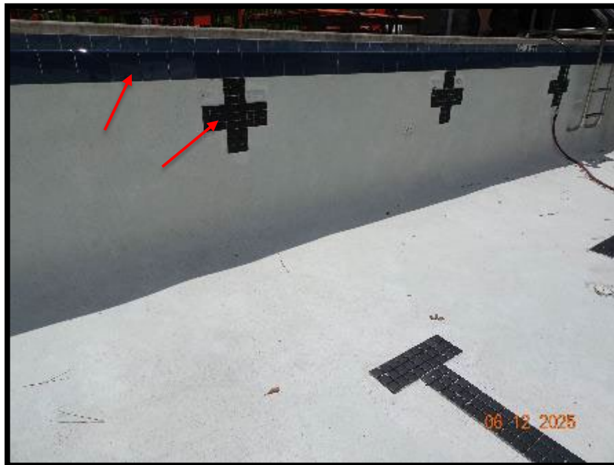
Photo 8 View of replaced/repaired tile along skimmer ledge location.
