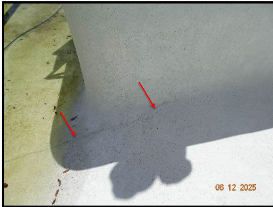
Photo 5 Close-up view of formed crack along reentrant corner.
