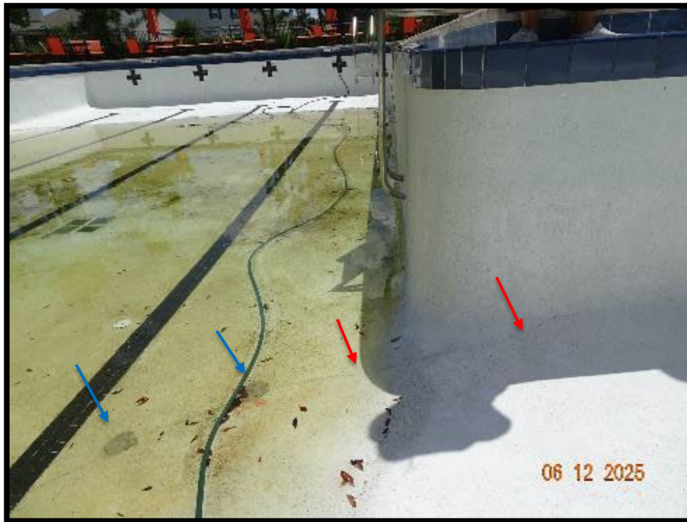
Photo 3 View of reentrant corner area of the pool where a crack was formed. Red arrows depict crack location. Blue arrows depict location of Core areas C1, and C5.
